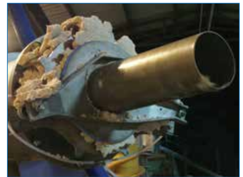
Tapioca processing (SEPCOM Industrial Vertical)
