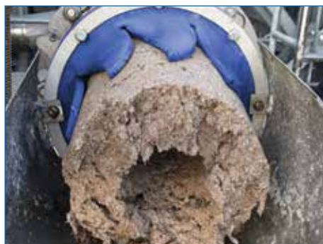
Paper mill (SEPCOM Industrial Horizontal)
